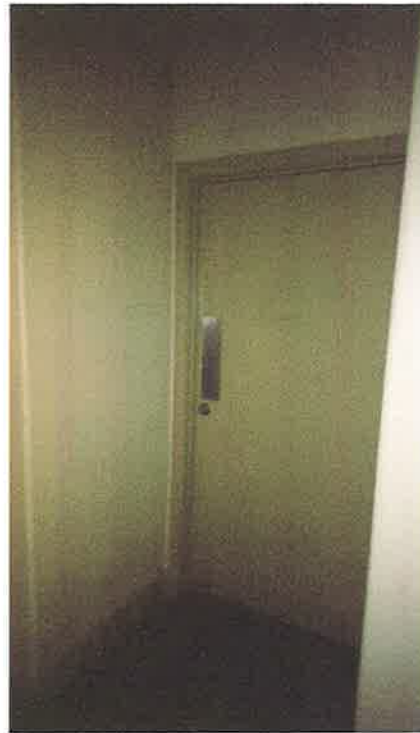
Women's Bathroom now a storage
